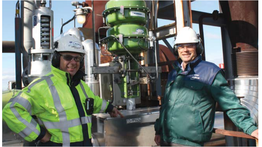
Rob Fok, Projectleider BioMCN - Marc Westerhuis, Sales Engineer Klinger BV
