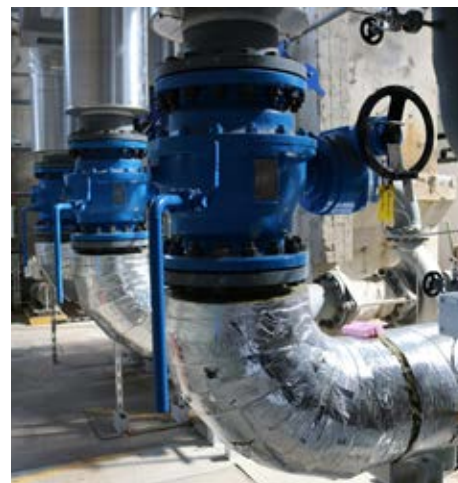
KLINGER valves in Central Europe's largest heat pump
