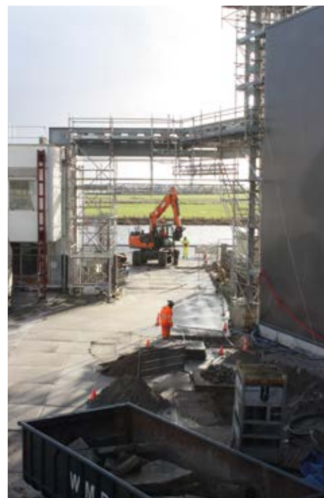
Construction time: The plant expansion was carried out on a step-by-step basis
