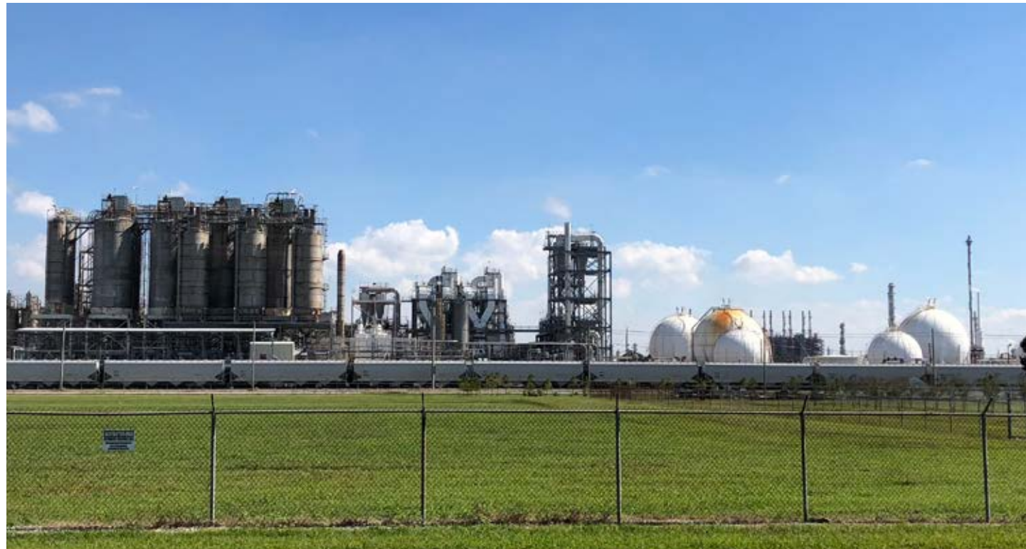
Westlake Chemical operates a polyvinyl chloride plant in Baton Rouge, Louisiana
