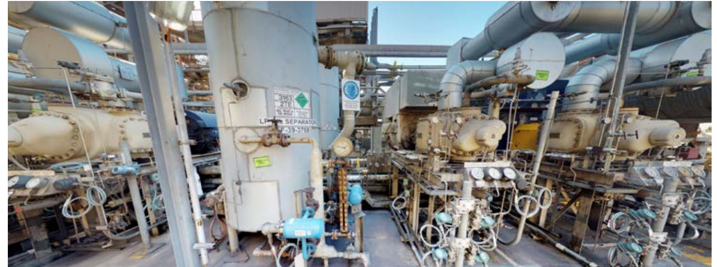
In 3D: A customer plant, ready for inspection in ATMECO's Component Integrity Management System (CIMS)
