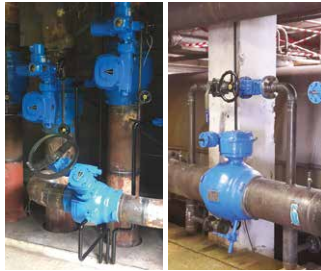
Heating supply and return
