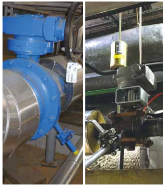
Isolation of pumps
