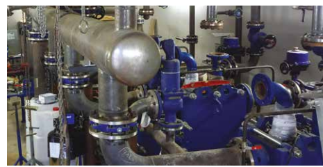
Sub-station (at the heat-exchanger inlet)
