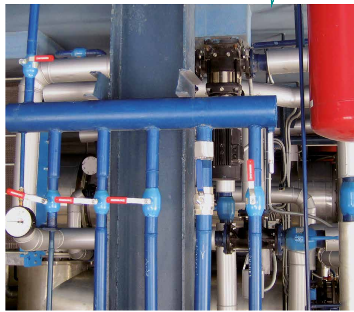
Sub-station (at the heat-exchanger outlet)
