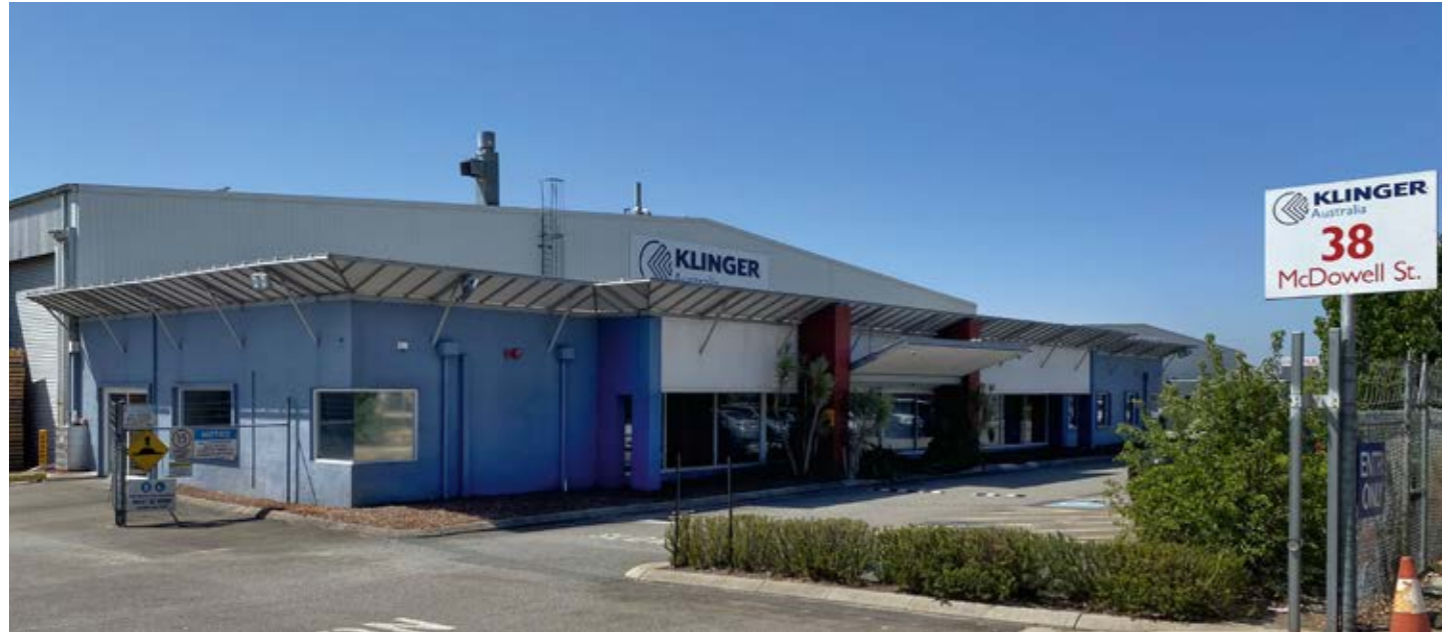
KLINGER Australia's plant in Western Australia
