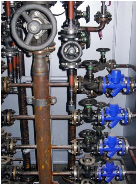
KLINGER Piston valve Type KVN
